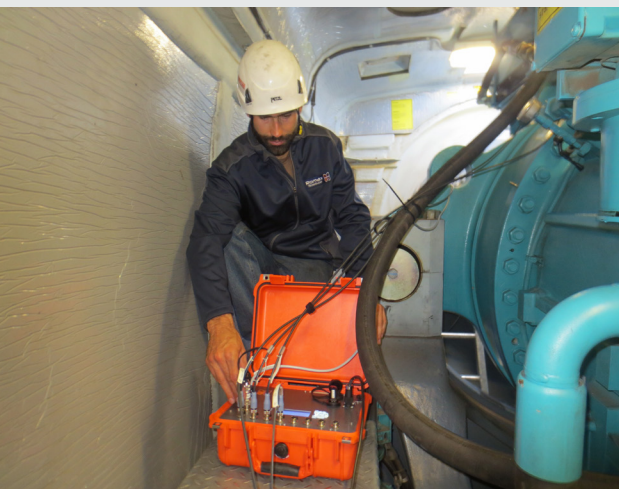
Romax engineer installing PVS equipment
